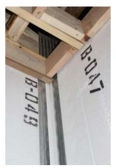
Figure 3: Numbered panels for easy assembly and raised heel construction
