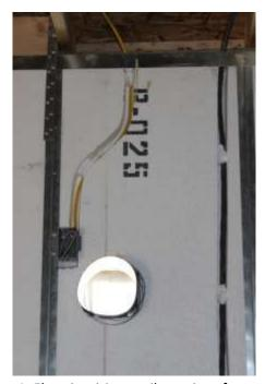
Figure 4: Electric wiring easily cut into foam panel
